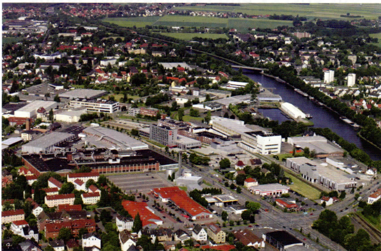
Melitta's Minden facility has both a paper mill and converting plant
