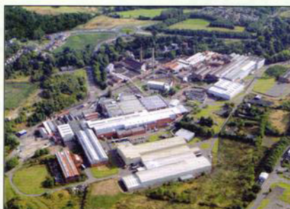
Tullis Russell at Markinch, where the biomass power plant will be built
